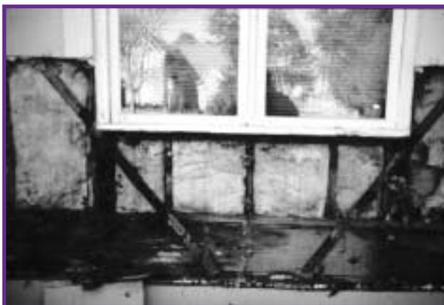
**Mold and decay are the result of moisture that accumulated in this wall.**
